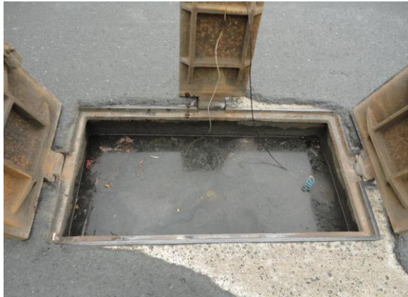
Difficulty in reading meters due to flooded chambers
