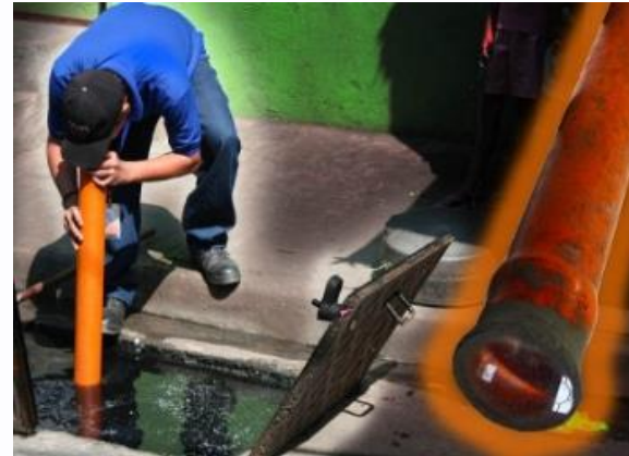
Meter reading using an improvised tool when chamber is flooded
